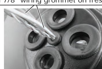
Route heavy gauge orange and white wires through 7/8" wiring grommet on fresh air cap
