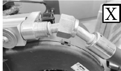
Improperly Seated O-ring Land
