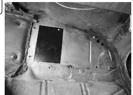
OEM Insulation Removed
