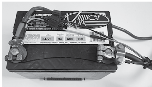
Completed Installation Shown
